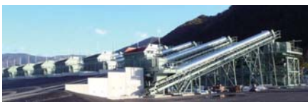
2011. Salt removal Plant Iwate - Ohfunato City
