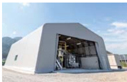
2013. Biogas pilot plant Iwate - Ohfunato-City
