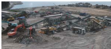
2011. Secondary screening plant Iwate Ohfunato-City
