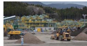
2013. Wet/dry sediment screening plant Iwate Rikuzentakada-City
