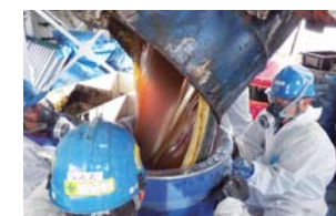
Removal of materials from decayed drums
