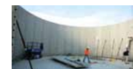
Assembling a methane fermentation tank
